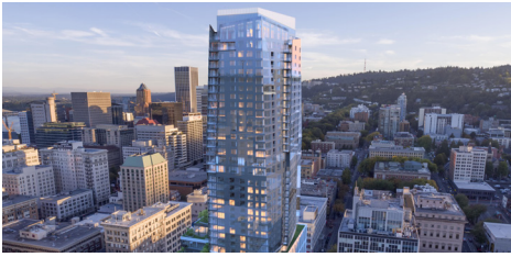
Block 216/Ritz-Carlton Tower 812 SW Washington St
