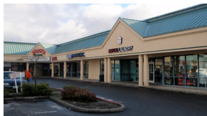
EASTWAY CENTER Renton, WA
