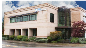
GBC BANK BUILDING Shoreline, WA
