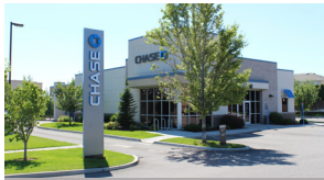
CHASE BANK Lynnwood, WA
